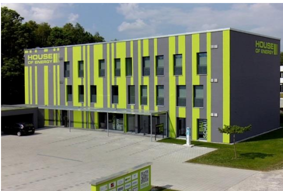
The world's first Passive House Premium building, located in Kaufbeuren in Bavaria. Photo: Airoptima
